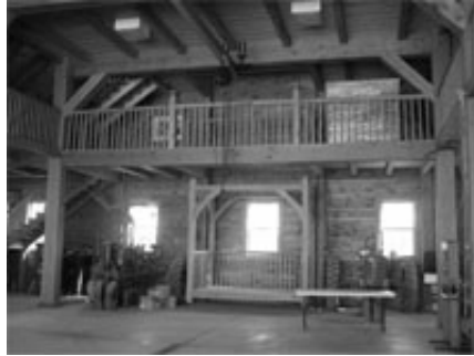
Inside look including the elevator and wide center aisle.
