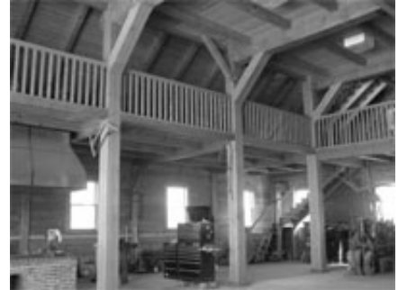
Typical beams and structure joints.
